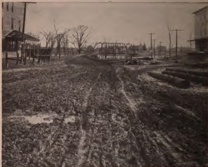
A Wayne County Road Before Improvement.
